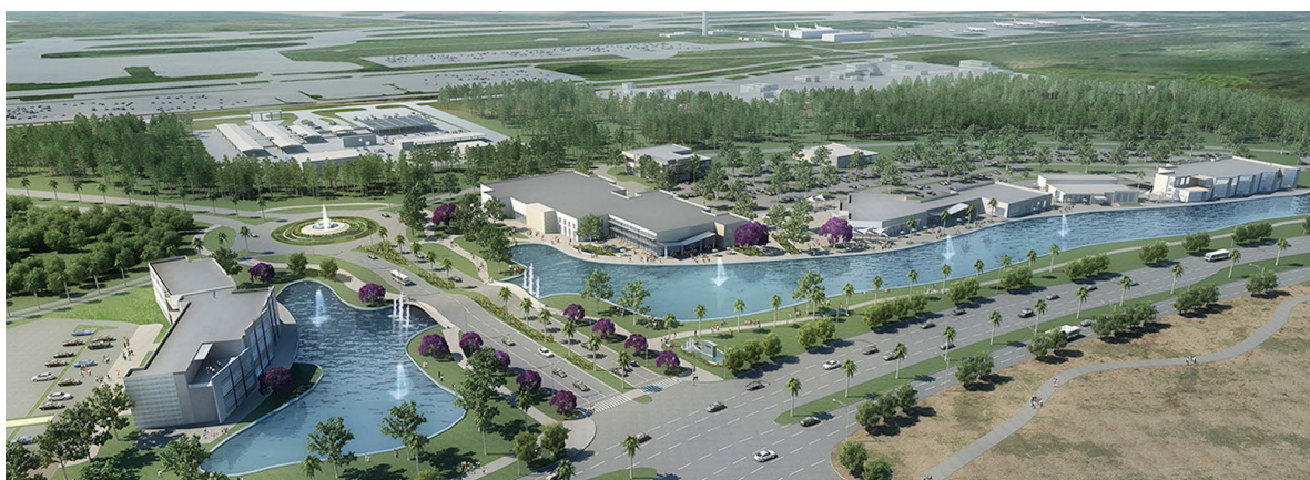
COURTESY RENDERING — Skyplex, a 1,150-acre business park adjacent to Southwest Florida International Airport, wants to lure Class A office users.
